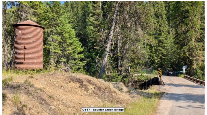
GT17 - Boulder Creek Bridge
