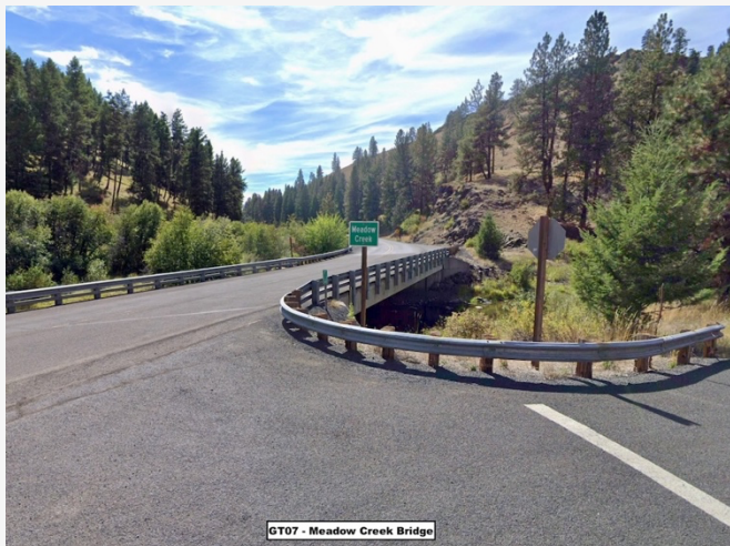
GT07 - Meadow Creek Bridge
